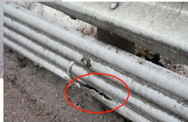
Damages from the snow plough after the first winter
